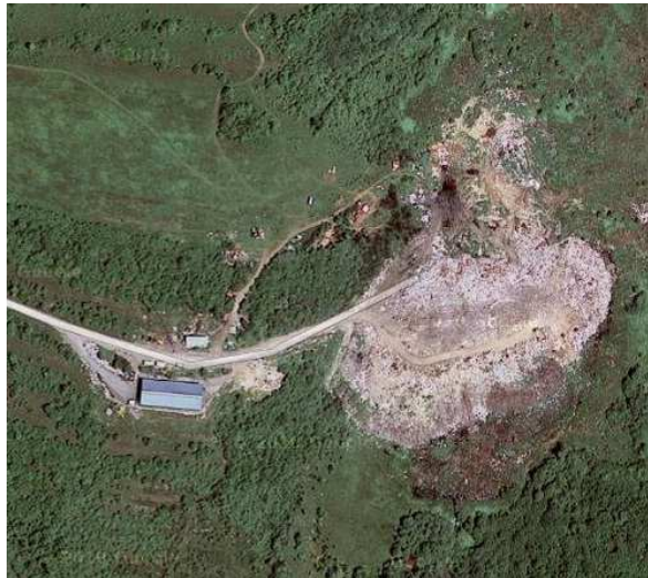
Figure 2.1 General View of Gabrovo Landfill
