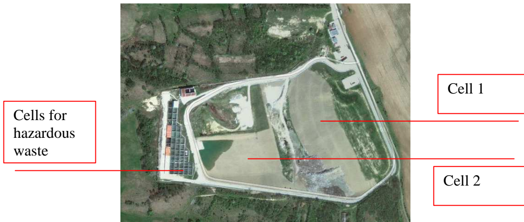
Figure 2.5 General View of Sevlievo Landfill
