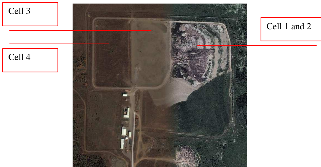
Figure 2.3 General View of Montana Landfill
