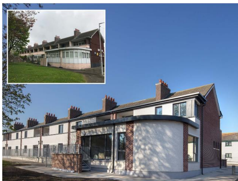
Figure 13. Case study in Ireland, St. Brigid's Pre & Post Renovation
