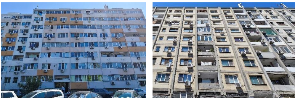
Figure 3: Examples of large residential buildings with installed air conditioners
